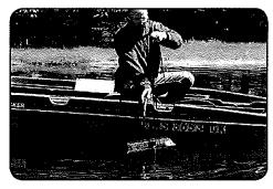
Use rope looped around diffuser to assist lowering assembly to pond bottom.
