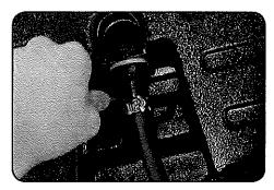
Slide hose clamp back over tubing and fasten with regular screwdriver or nut driver.
